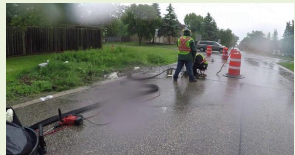
Fig.3 precast slabs under sealed with polyurethane foam
